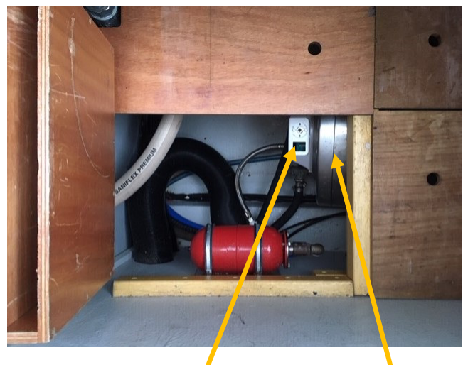
2. Location of thermal cut out switch and Calorifier
