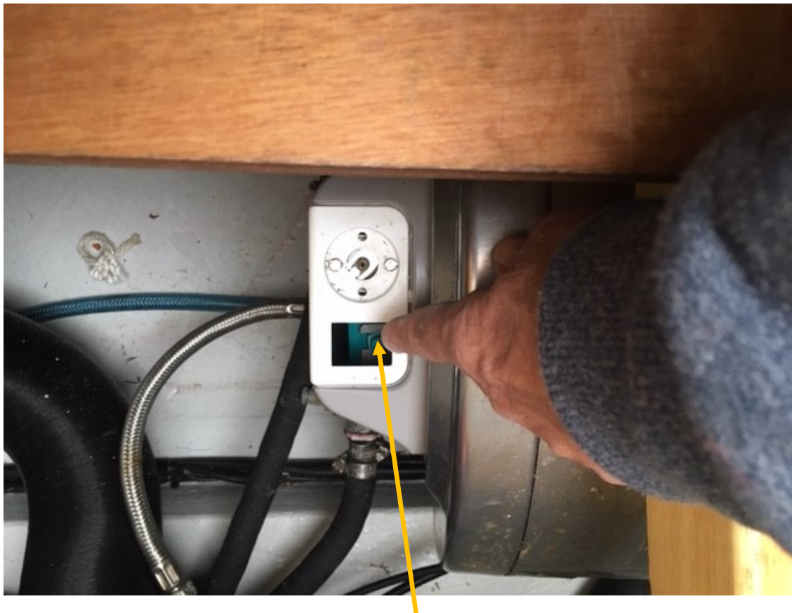
Thermal Cut Out Switch for Calorifier
